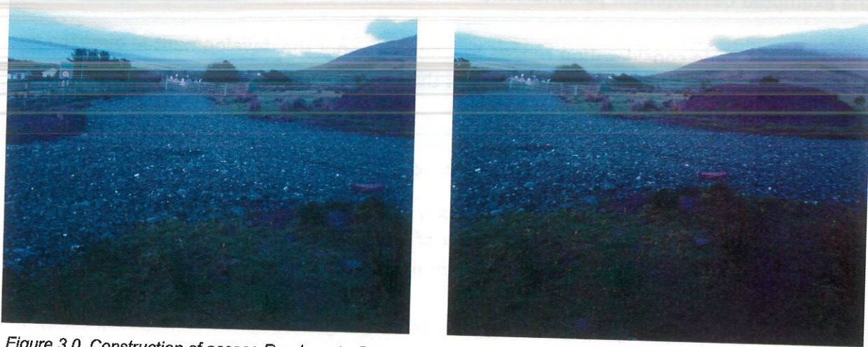
Figure 3.0 Construction of access Roadway to Compound
